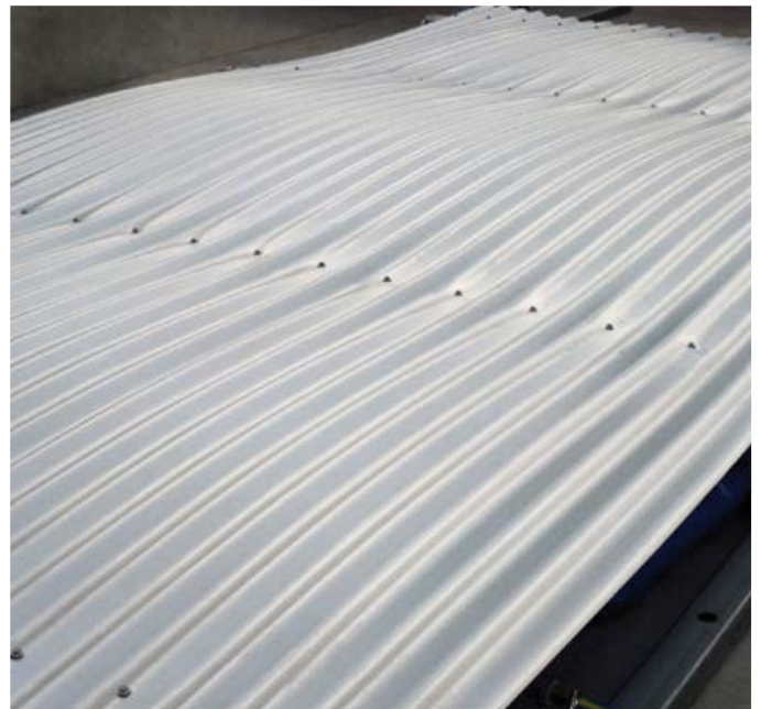
Roof Pressure Test
